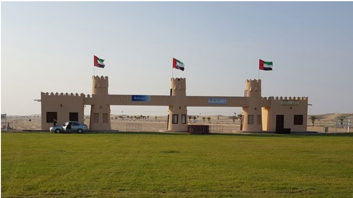
1.- The brand new portico where starts and finishes take place. The design is new with the photographers' office on the right and a ride management office mainly dedicated to on course weighing on the left.
